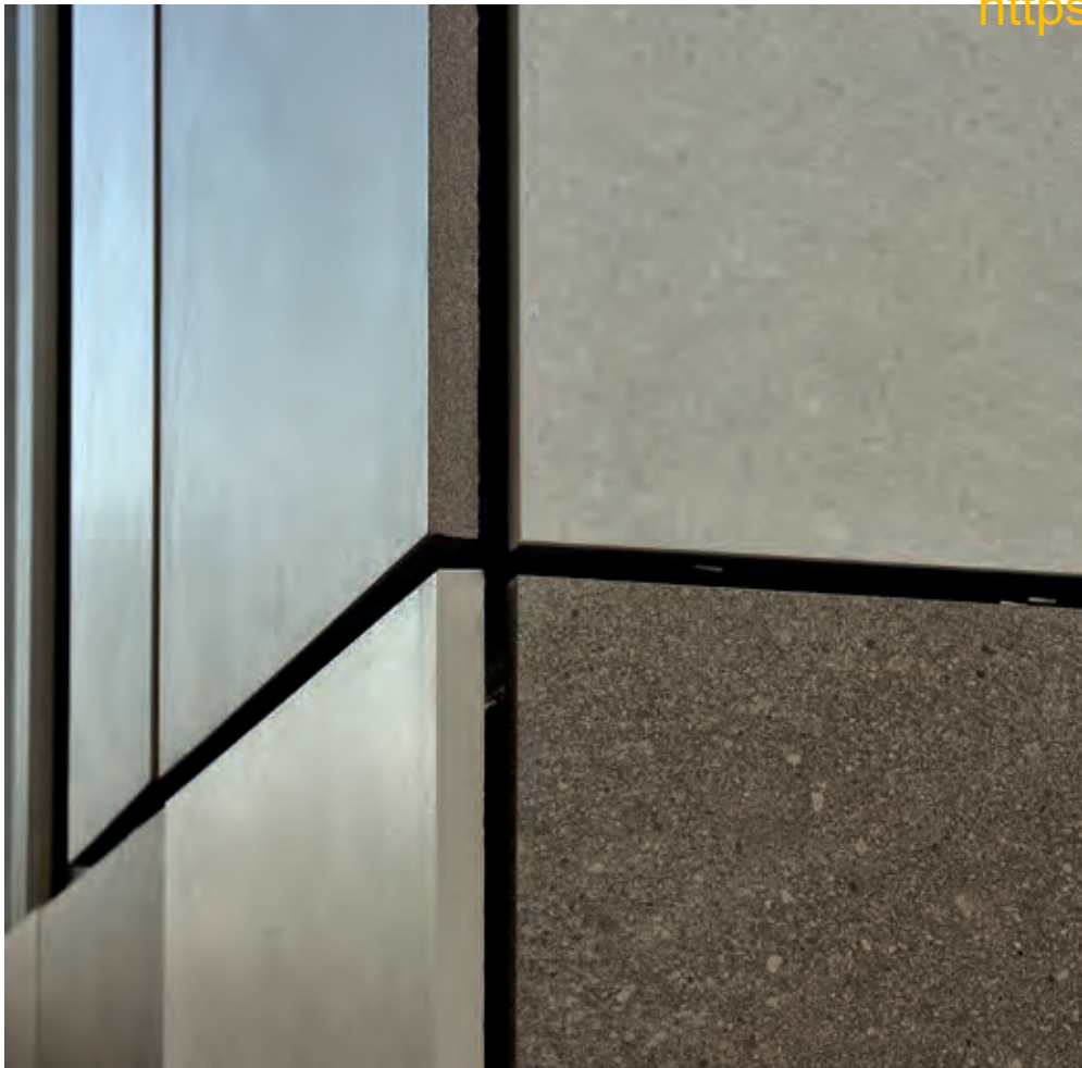
Project: Azienda Isocell Photos: Luciano Busani
