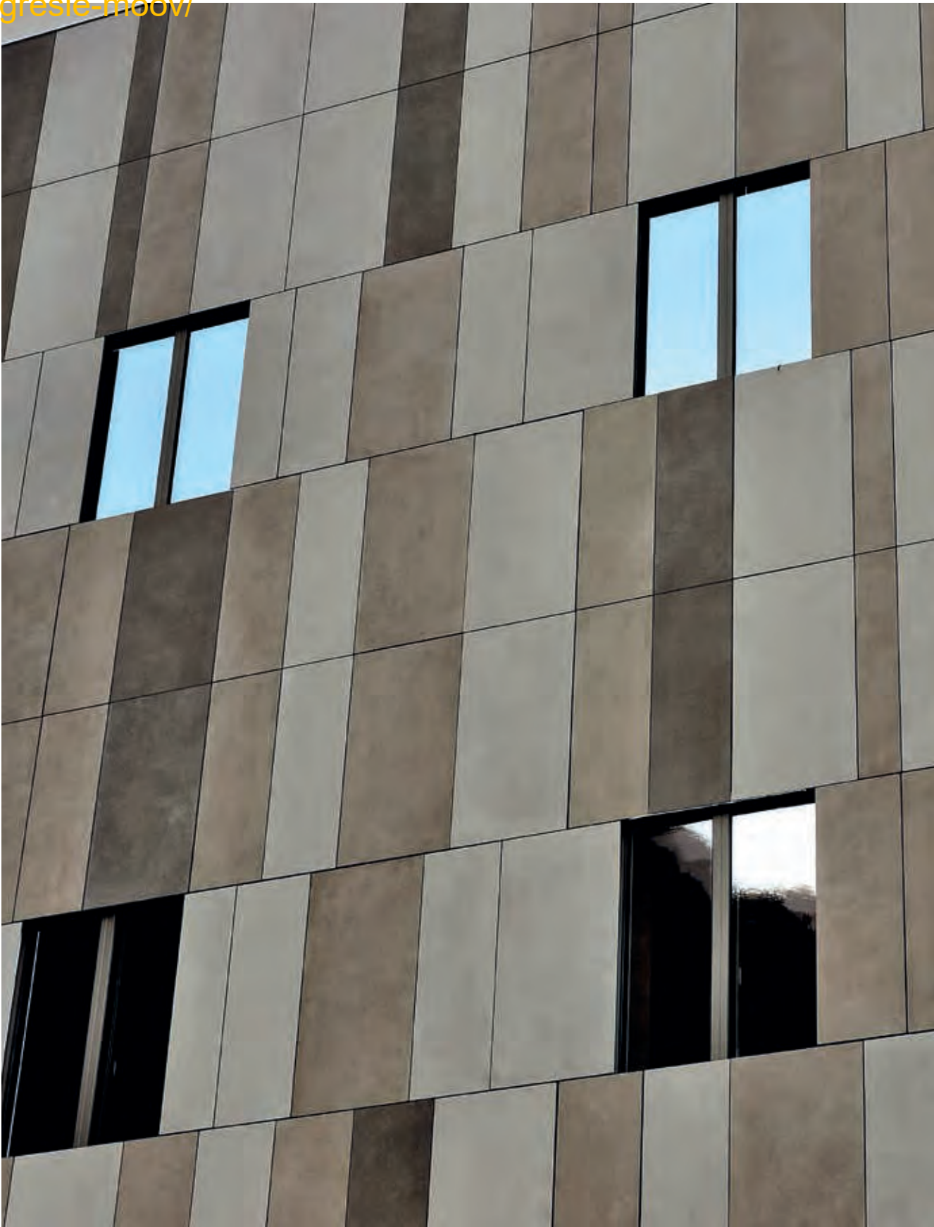
Project: Azienda Isocell Photos: Luciano Busani
